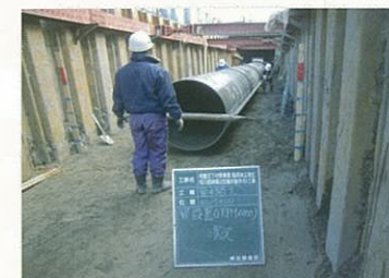
(工事中)FRPM管φ1100mm
